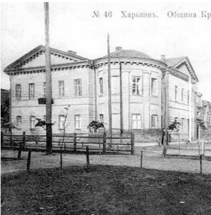
Fig.4 The building of Kharkov Red Cross hospital (up to 1912).
